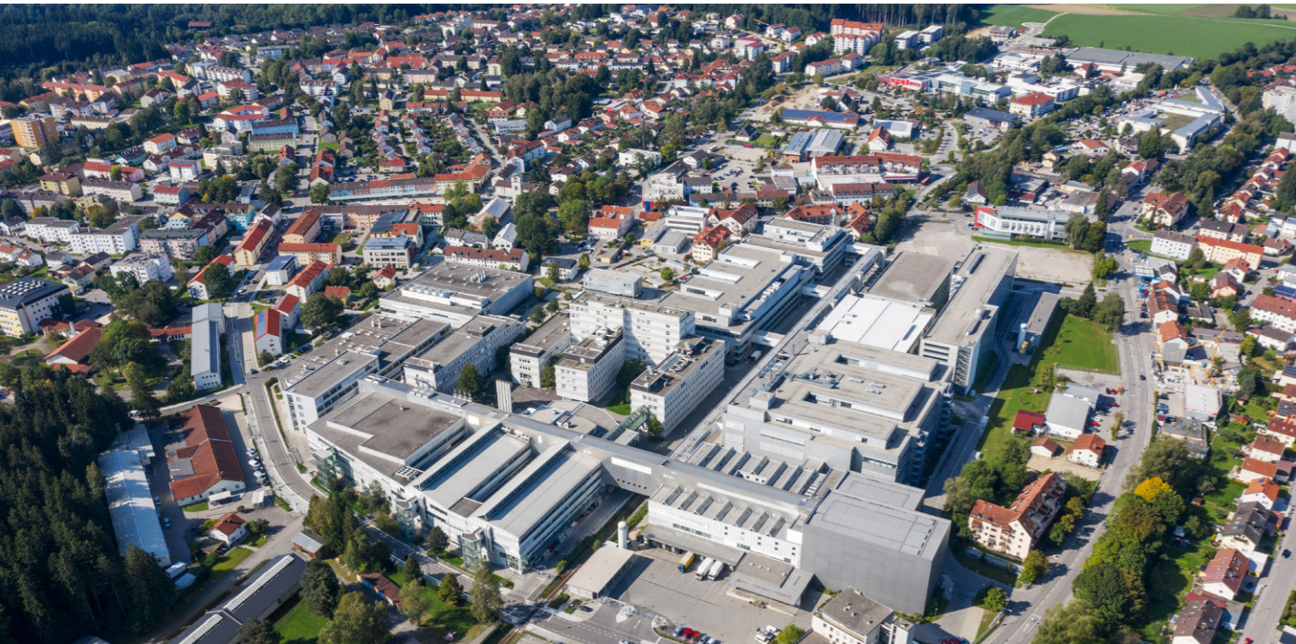
Head office and main plant in Traunreut
